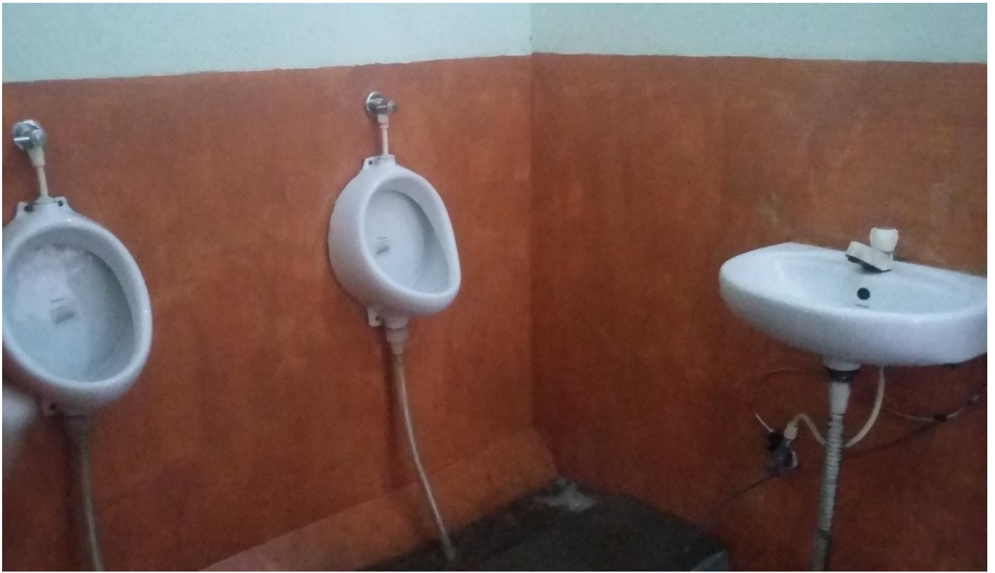
Boys Toilet Room
